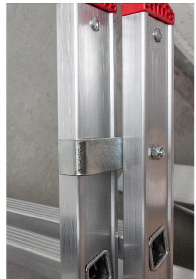
In combination ladders, the top guides are equipped with hinges (see photos below) that allow the ladder to be used as a trestle ladder. It is important that the hinge pin is correctly placed in its slot when the ladder is used as a trestle ladder.
